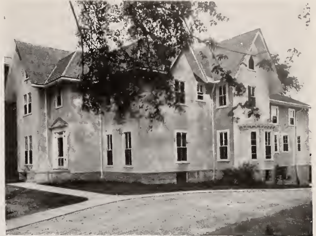
Wonderful transformation of forty-five year old wood frame house to modern stucco residence. \frac{3}{8} " Hy-Rib Lath was applied directly to the old siding without the use of furring strips. David Stott Estate, 1700 E. Jefferson Ave., Detroit, Mich. John Shea, Plastering Contractor.
