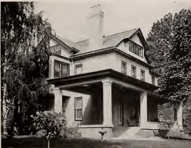
Residence of Arnold Kaichen, Cincinnati, Ohio. An Old Wooden House Transformed into a Modern, Permanent Residence by Overcoating with Hy-Rib Lath and Stucco.
