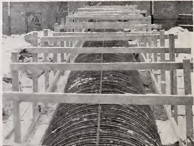
Hy-Rib passageway connecting buildings of Wayne County Insane Asylum, Eloise, Mich.
