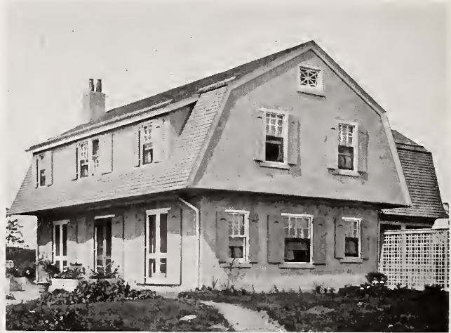
Hy-Rib Concrete Residence—Dr. Terriberry, Fisher's Island, N. Y. James Sweeney, Architect.
