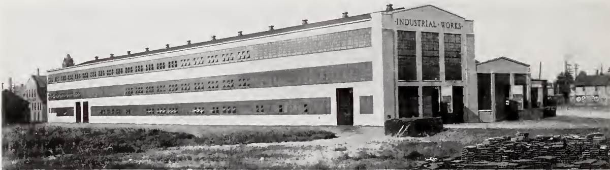
Hy-Rib Concrete Roofs and Sidings, Industrial Works, Bay City, Mich. Albert Kahn, Architect.
