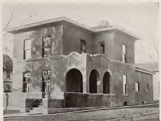
Hy-Rib Plastered with Cement Stucco. Residence of N. J. Spaulding, Ionia, Michigan.
