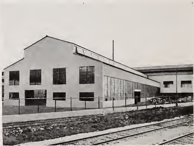
Hy-Rib Concrete Sidings, Mark Manufacturing Co., Evanston, Ill. Steel windows in walls and monitors furnished by Truscon Steel Co.
