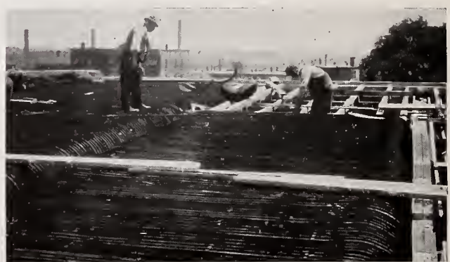
Arched Hy-Rib Floor—Union Street Ry., Boston, Mass.
