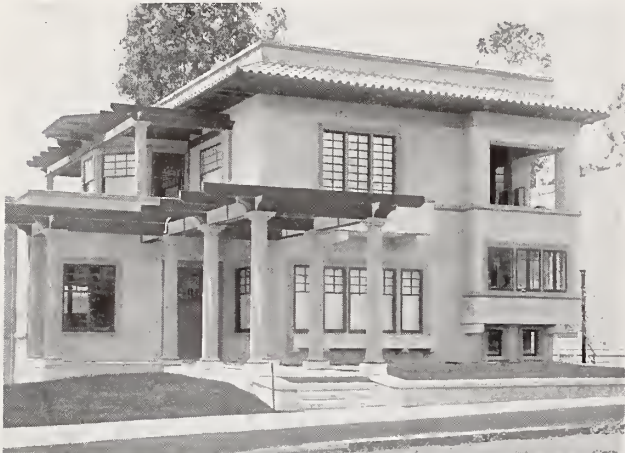
Hy-Rib Residence for Miss Alice Henck, Santa Barbara, Cal. Thomas Nixon, Architect.
