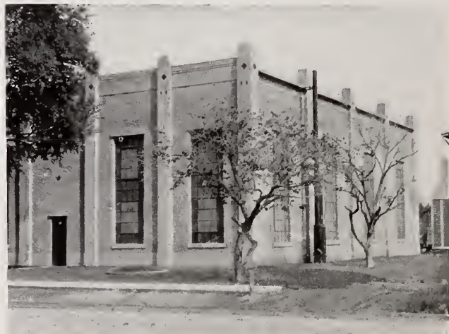
Hy-Rib Concrete Siding, Power House, Gainesville, Texas.
