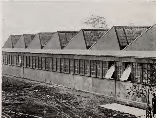
Hy-Rib Concrete Saw-tooth Roofs and Sidings. Jackson Cushion Spring Co., Jackson, Mich.
