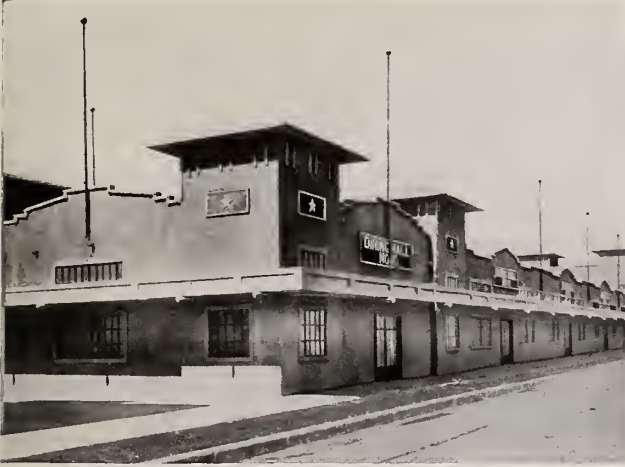
Texas State Fair Assoc., Dallas, Tex., Restaurant Row (500' x 44'). Hy-Rib Concrete Walls, Truscon Reinforced Concrete, Steel Windows and Doors.
