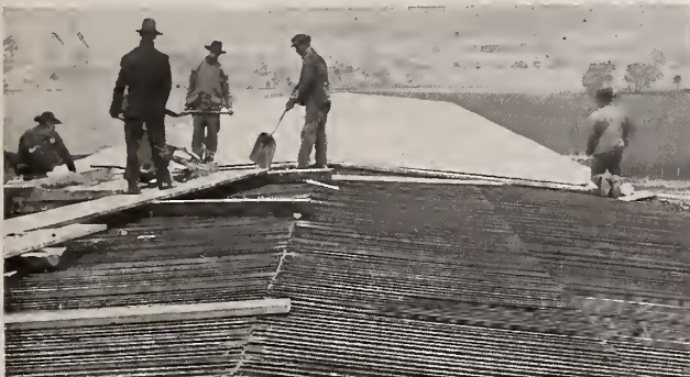
Hy-Rib Roof for Soft Foundry Building. American Car & Foundry Co., Berwick, Pa.
