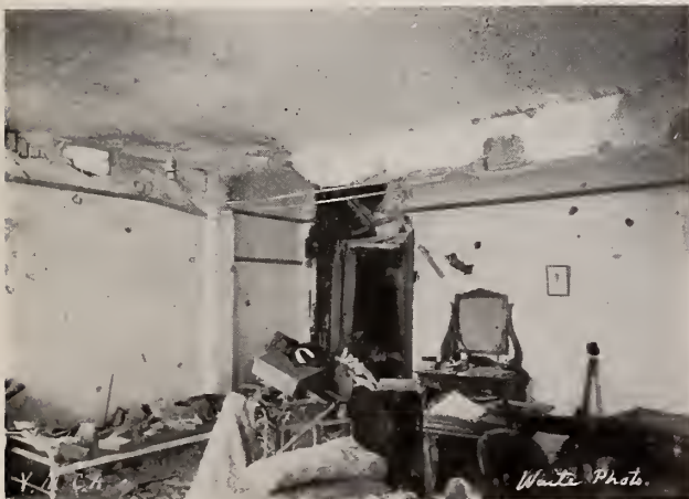
Two-inch Hy-Rib Partitions after bombardment with shot and shell in Y. M. C. A., Mexico City, February, 1913, illustrating the remarkable resistance of Hy-Rib Construction to severest shocks. Plastering holes at nominal cost are all the repairs necessary.
