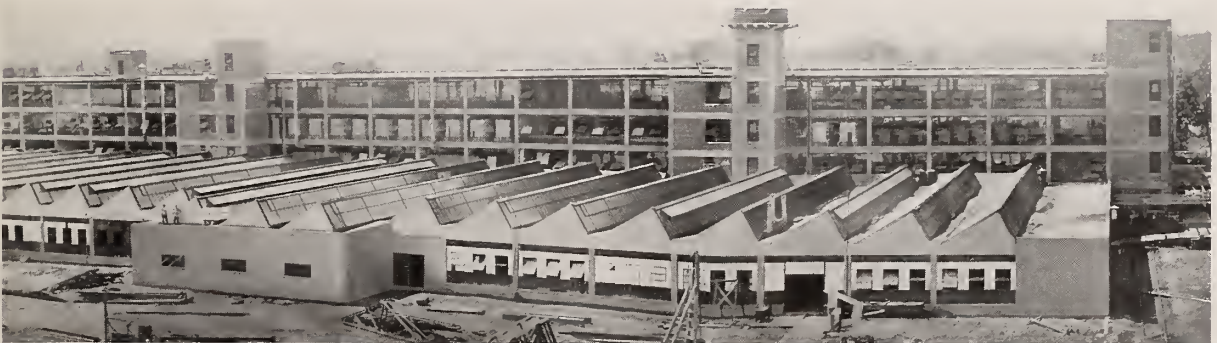
Hy-Rib Concrete Roofs and Sidings, Ford Motor Co., Detroit. Albert Kahn, Architect.
