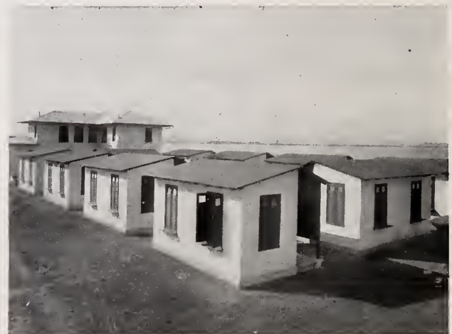
Quarantine Hospital Buildings, Porto Rico. Built of Hy-Rib Con- crete Construction.
