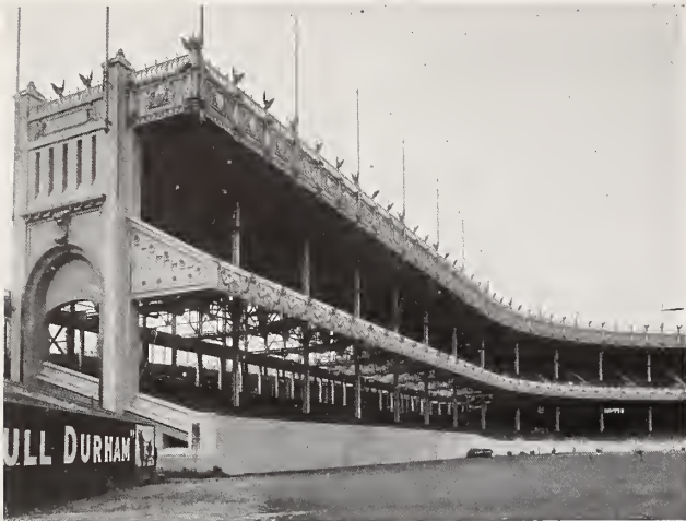
Polo Grounds, New York. Snare & Triest Co., Erectors. Hy-Rib used in all Sidings, Partitions, Ticket Booths, Railings, etc.
