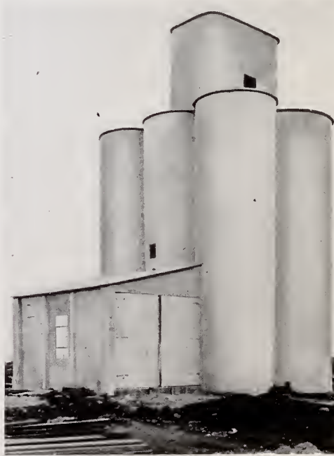
Hy-Rib Concrete Grain Tanks for the Independent Co-operative Grain & Mercantile Company, Stafford, Kansas. Many of this kind have been built by the Concrete Steel Machinery Co., Kansas City, Mo.
