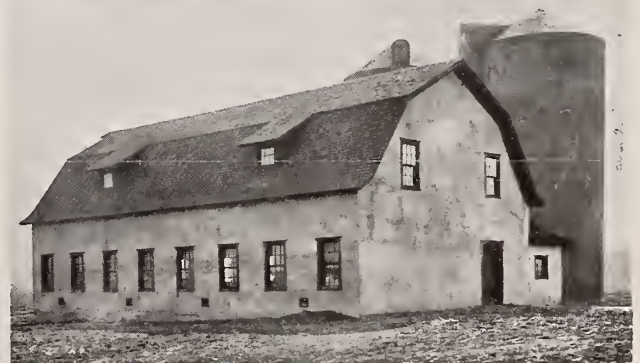
Hy-Rib Feed Barn and two Hy-Rib Silos. Espanore Farm, Lansing, Mich. Ex-Governor Osborne, Owner.
