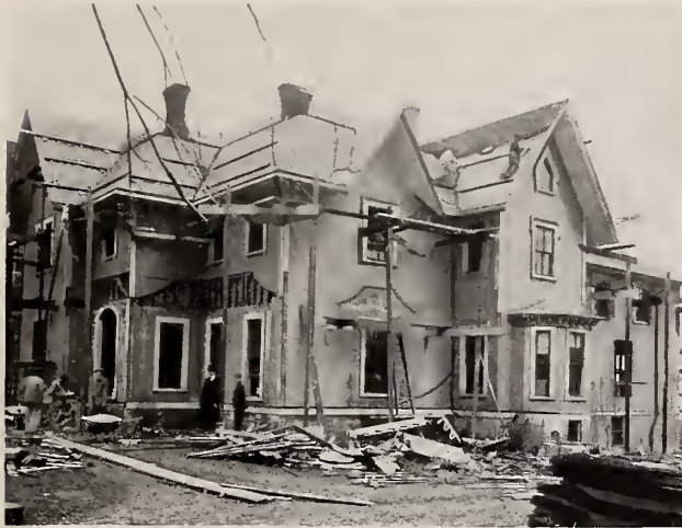
Wonderful transformation of forty-five year old wood frame house to modern stucco residence. \frac{3}{8} " Hy-Rib Lath was applied directly to the old siding without the use of furring strips. David Stott Estate, 1700 E. Jefferson Ave., Detroit, Mich. John Shea, Plastering Contractor.
