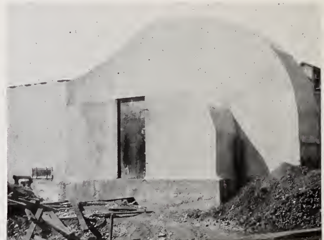
Fan House built of Hy-Rib Concrete. Birmingham Fuel Co., Birmingham, Ala.
