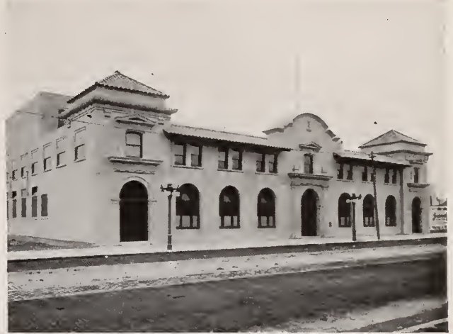
Sunset Publishing Co., San Francisco, Cal. Geo. W. Kelhane, Architect. The exterior concrete walls are built with Hy-Rib on wood studs.
