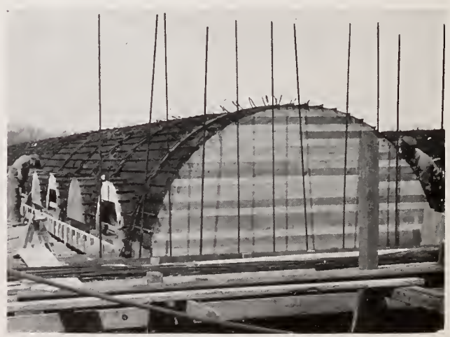
Roof of 1½" Hy-Rib, Fairview Mausoleum, Milwaukee, Wis.
