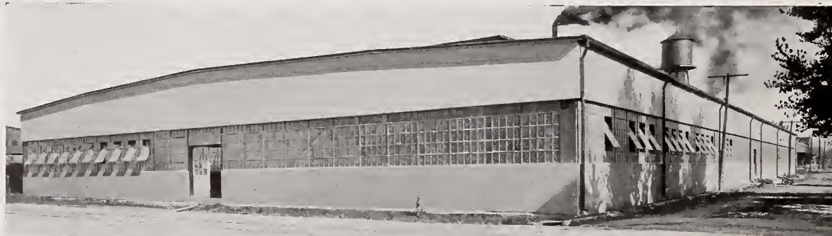
Hy-Rib Concrete Sidings, Favorite Stove & Range Co., Piqua, Ohio. William E. Russ, Architect.
