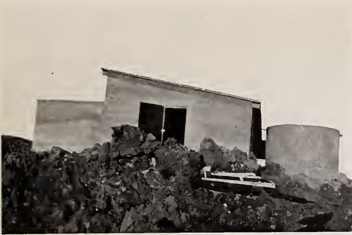
Hy-Rib Concrete Rest-House at Kaleakala Crater, Hawaiian Islands. Hy-Rib Concrete Tank at right.
