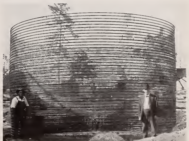
Water Tank (Hy-Rib), Jefferson Powder Co., Birmingham, Ala. Hy-Rib bent to exact curve in our shops.
