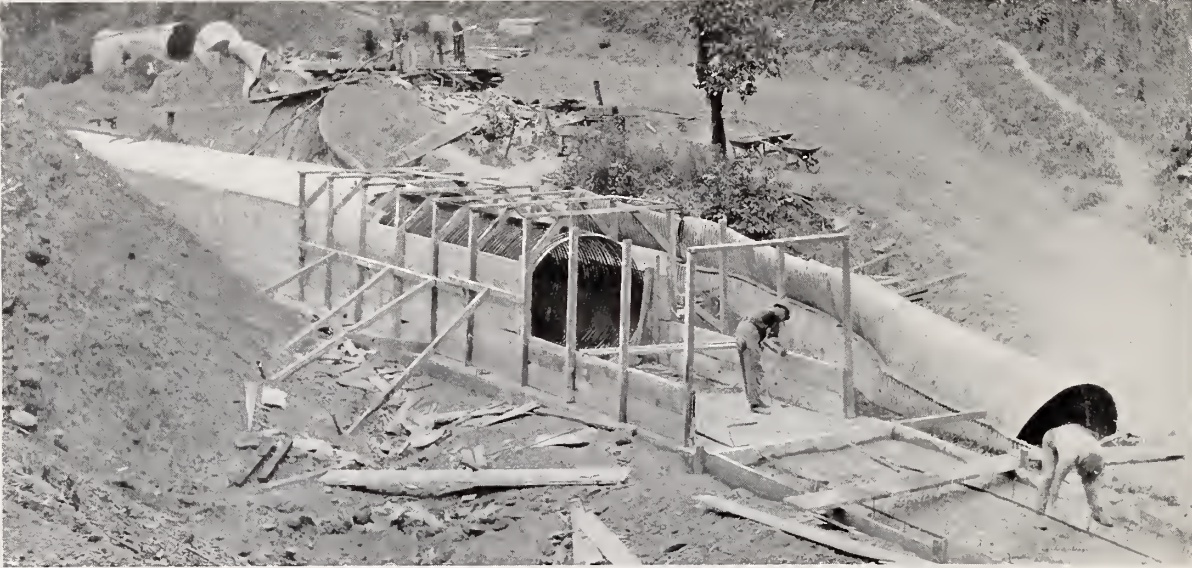
Hy-Rib Concrete Culvert, Charleroi Mine, Carnegie Coal Co., W. Monessen, Pa.
