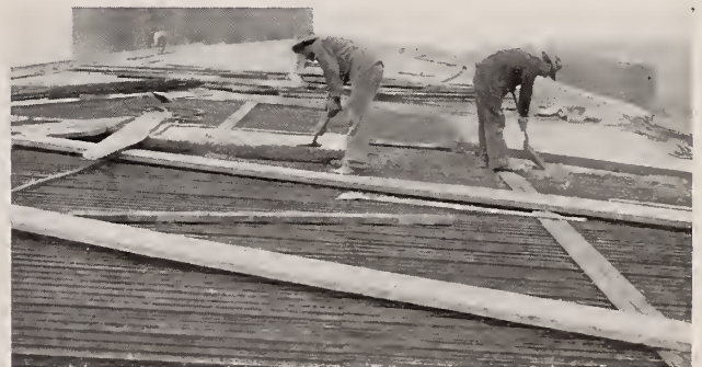
Hy-Rib Roof for Soft Foundry Building. American Car & Foundry Co., Berwick, Pa.
