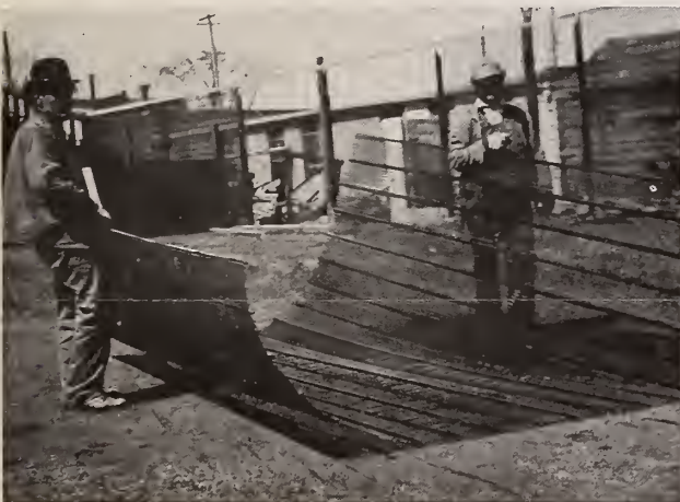
Hy-Rib Concrete Fence, Minneapolis Ball Grounds. Hy-Rib sheets are united by punching and placed a panel at a time. Note the great saving in labor by the use of Hy-Rib and this method of handling.
