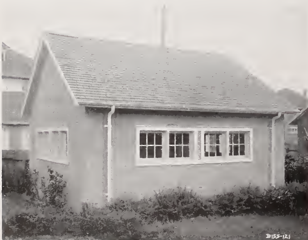
Stucco Garage of S. M. Fechheimer, Highland Park, Mich. \frac{3}{8} " Hy-Rib Lath on Wood Studs, Stuccoed and Back-plastered.
