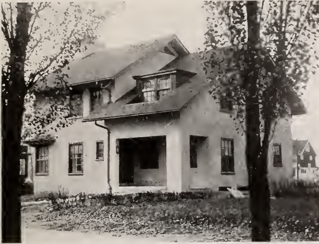
Stucco on Hy-Rib Metal Lath. Residence of Harvey Whipple, Detroit, Michigan.
