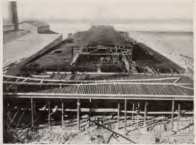
Hy-Rib Roof ready for concreting, Hayden Pump Co., Quincy, Ill. No forms required.
