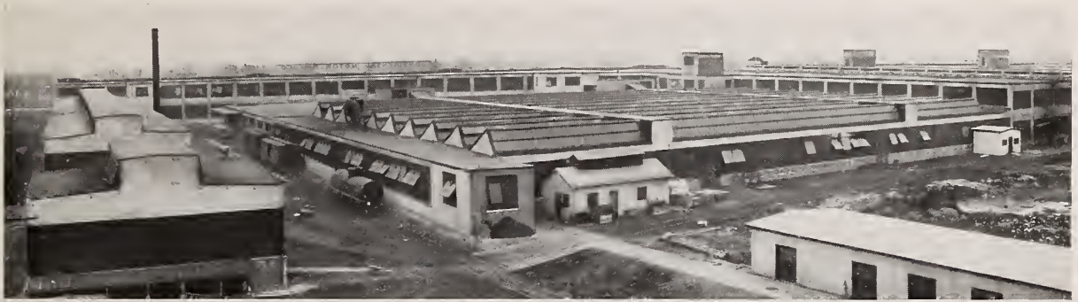
Hy-Rib Concrete Roofs and Sidings, Continental Motor Corp., Detroit, Mich. Albert Kahn, Architect.
