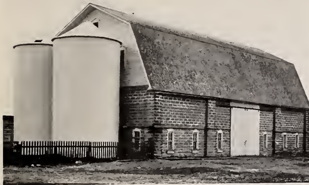
Two 14'x30' Hy-Rib Concrete Silos on the McBride Farm, Burton, Mich.
