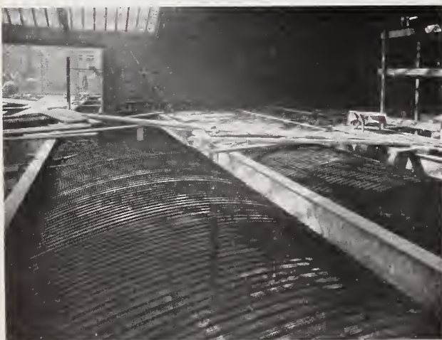
Westgate Common Mills, London, England. Arched Hy-Rib before application of concrete.
