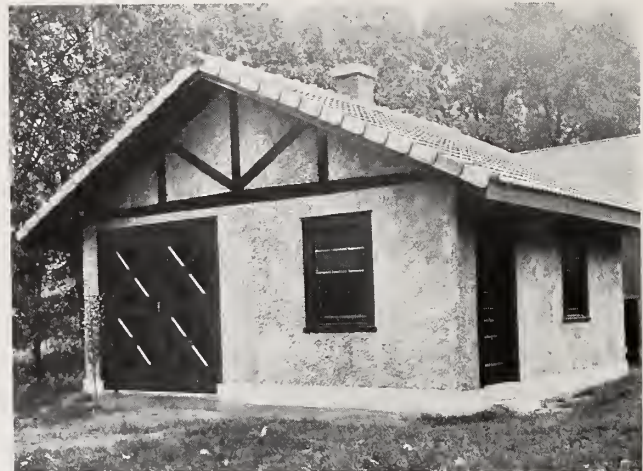
Hy-Rib Concrete Garage for Luke Cates, Webster Groves, Mo.
