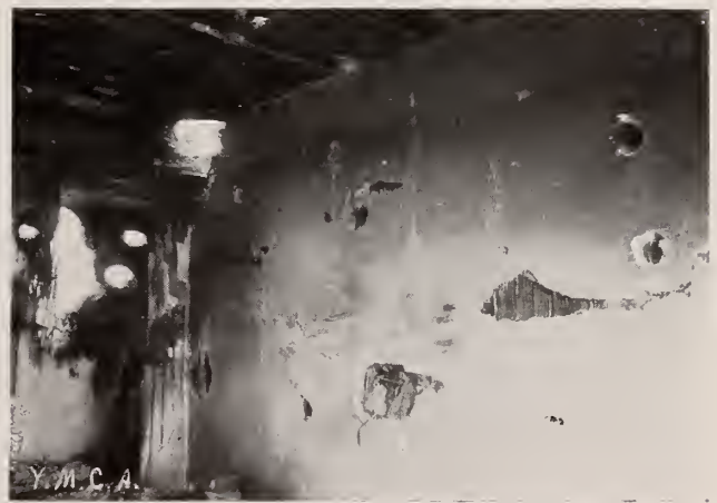
Two-inch Hy-Rib Partitions after bombardment with shot and shell in Y. M. C. A., Mexico City, February, 1913, illustrating the remarkable resistance of Hy-Rib Construction to severest shocks. Plastering holes at nominal cost are all the repairs necessary.
