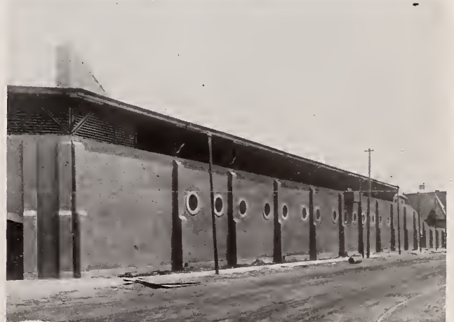
Hy-Rib Concrete Fence, Minneapolis Ball Grounds. Hy-Rib sheets are united by punching and placed a panel at a time. Note the great saving in labor by the use of Hy-Rib and this method of handling.
