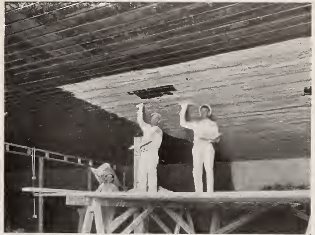
Hy-Rib Ceilings, Bremer Arcade Building, St. Paul, Minn. Buechner & Orth, Architects. Wm. Poppenberger & Sons, Plastering Contractors. Note method of suspending Hy-Rib without use of small channels. Note also heavy first coat of plaster.
