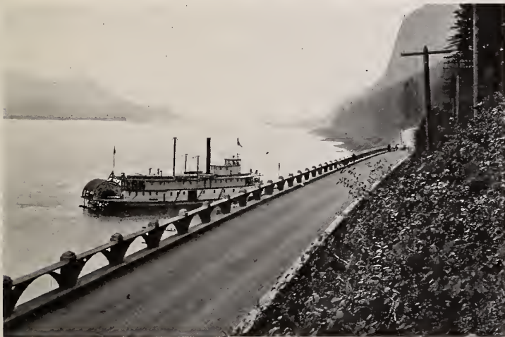
Hand Railing of plastered Hy-Rib on mountain-side viaduct, Columbia River Highway, Oregon.
