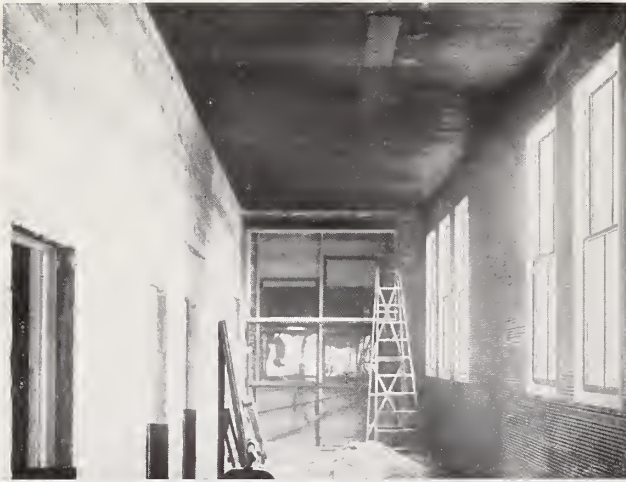
Hy-Rib Lath for Furring, Ceilings and Partitions. Grace Hospital, Detroit, Mich.
