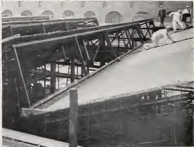
Hy-Rib Concrete Sawtooth Roofs and Side Walls, Western Sugar Refining Co., San Francisco, Cal.
