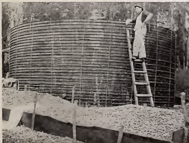
25,000-gallon Concrete Reservoir, City of Monroe, Ore. Hy-Rib Concrete Construction.
