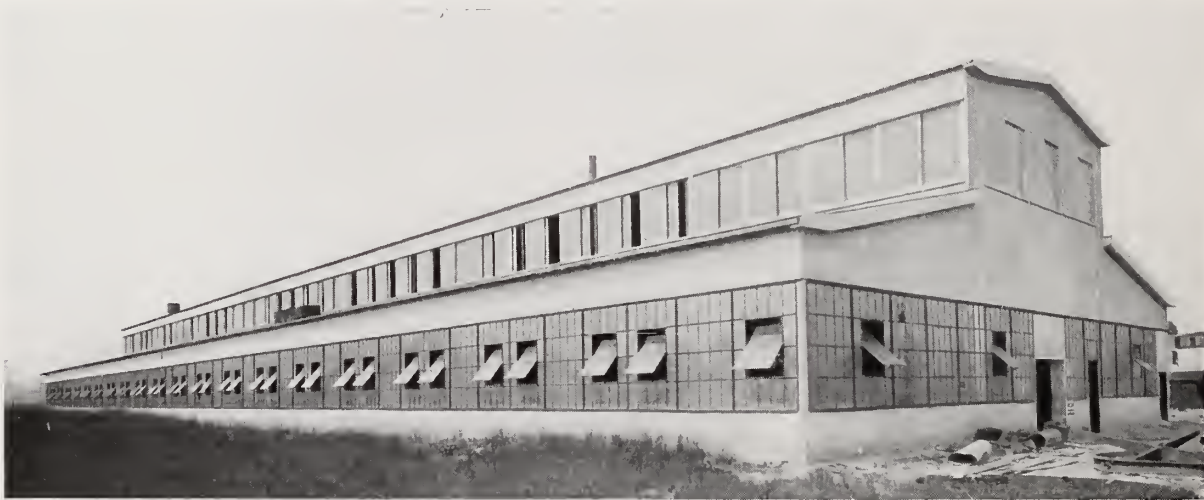
Hy-Rib Concrete Sidings and Steel Windows by Truscon Steel Co. Columbus Machine & Tool Co., Columbus, O.
