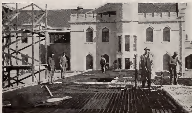
K. of P. Orphanage, Weatherford, Texas. Hy-Rib Floor ready for concreting.
