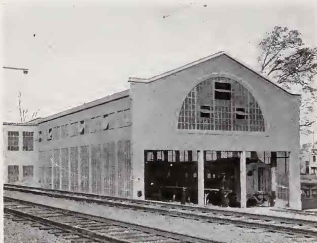
Coach Repair Shop, N. Y., Westchester & Boston R. R., New York. Hy-Rib Concrete Sidings. Steel Windows by Truscon Steel Co.
