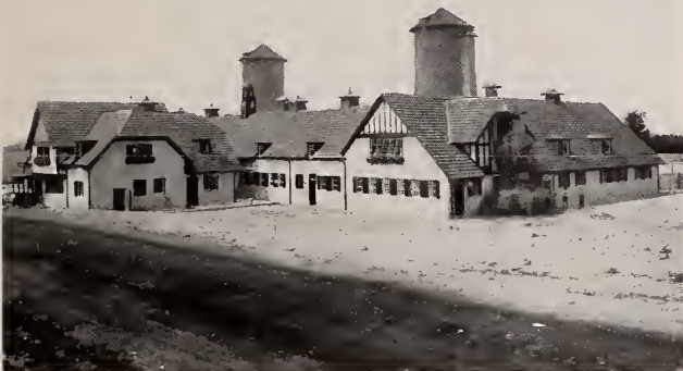
"Wabeek Farm," Birmingham, Mich. James Couzens, owner. Creamery and Dairy Barn of Truscon Reinforced Concrete. Hy-Rib Used for Concrete Silos, Fences and Partitions.
