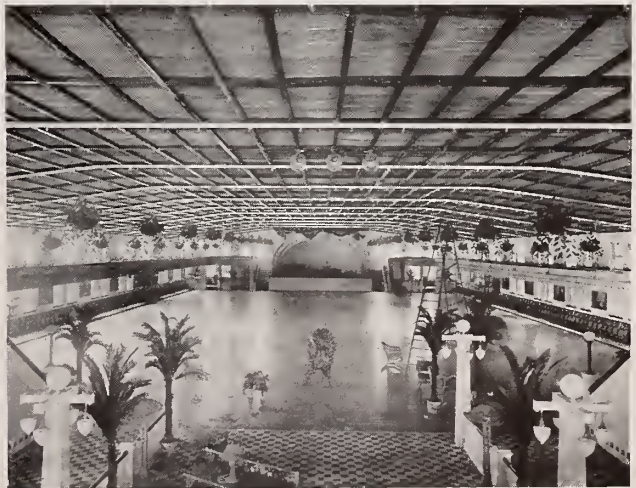
Guyon's Dancing Academy, Chicago, Ill. 1-A Hy-Rib Lath in Ceiling.
