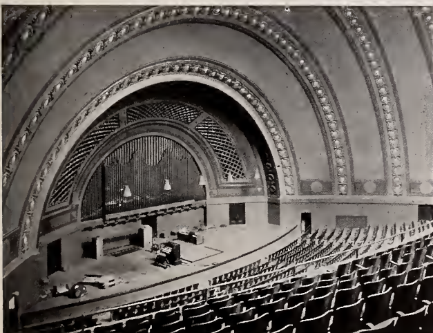
Hy-Rib Lath Ceilings. Hill Memorial Hall, University of Michigan, Ann Arbor, Mich. Albert Kahn, Architect.
