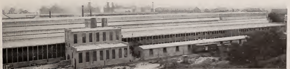
Hy-Rib Concrete Roofs, International Harvester Co., Springfield, O. De Vore-McGormley Co., Engineers.
