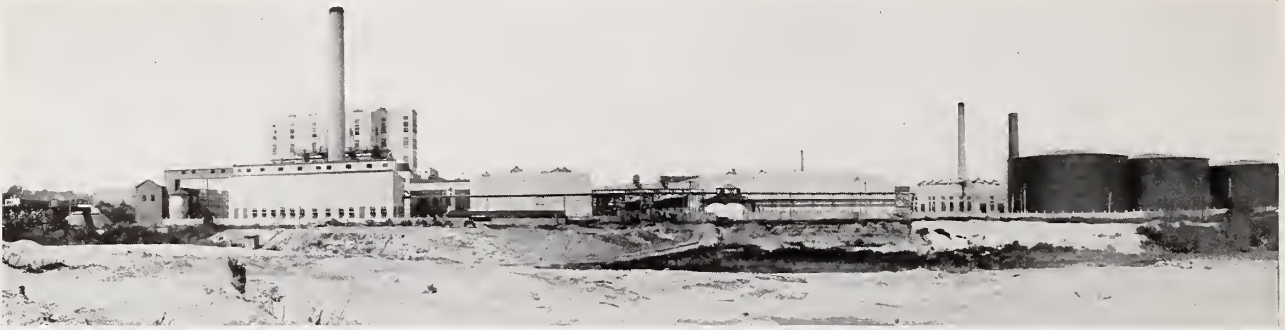
General Panoramic View of Curtis Bay Distilling Plant, Curtis Bay, Md. Hy-Rib Concrete Side Walls Used Throughout.
