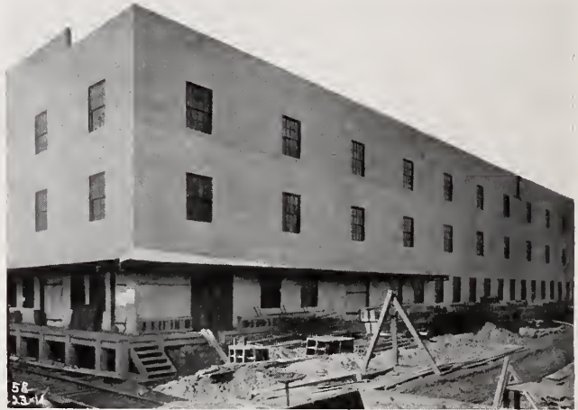
Cooperage Building, Curtis Bay Distillery. Hy-Rib Concrete Reinforcement for Walls.
