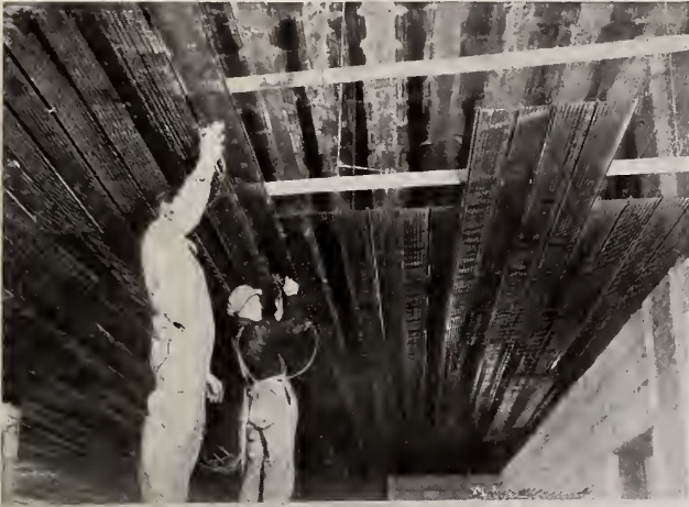
Hy-Rib Ceilings, Bremer Arcade Building, St. Paul, Minn. Buechner & Orth, Architects. Wm. Poppenberger & Sons, Plastering Contractors. Note method of suspending Hy-Rib without use of small channels. Note also heavy first coat of plaster.
