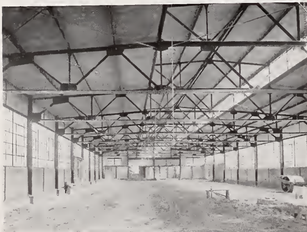
Barry Mfg. Co., Muscatine, Ia. Hy-Rib Concrete Sidings and Roofs. Truscon Steel Windows.
