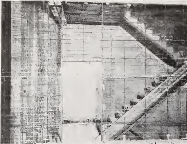
\frac{3}{8} " Hy-Rib Lath in Conrad-Windisch Bldg., Cincinnati, Ohio. Channels spaced 20" to 26" centers. Kruckmeyer & Strong, Architects. Mr. Bunyon, Plastering Contractor.
