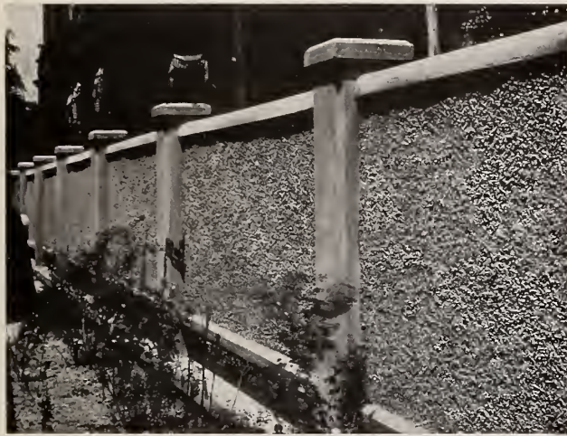
Hy-Rib Fence, E. J. Smith, Detroit, Mich. Note fence is open below.
