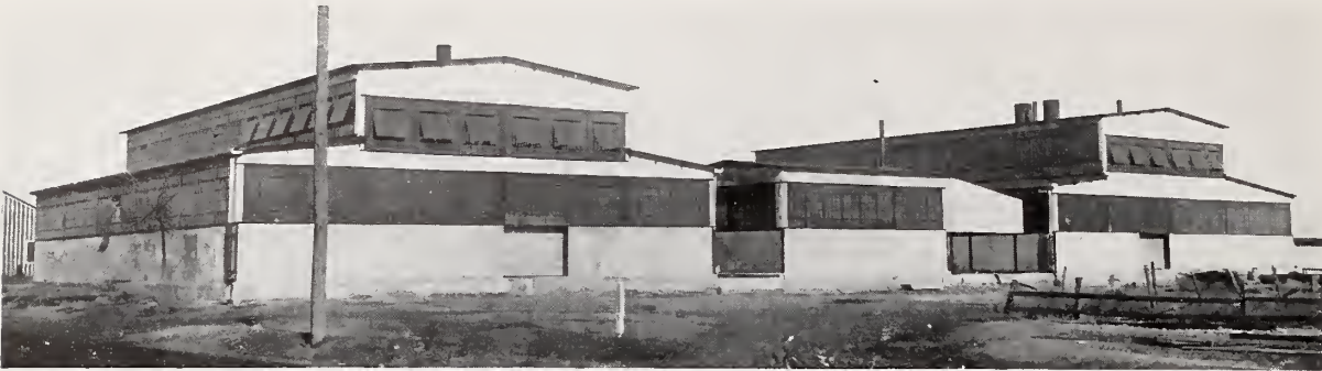
American Well and Prospecting Co., Corsicana, Texas. Hy-Rib Roofs and Sidings. Steel Windows Furnished by Truscon Steel Co.
